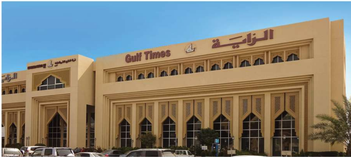
Project: Al Raya Newspaper Building
